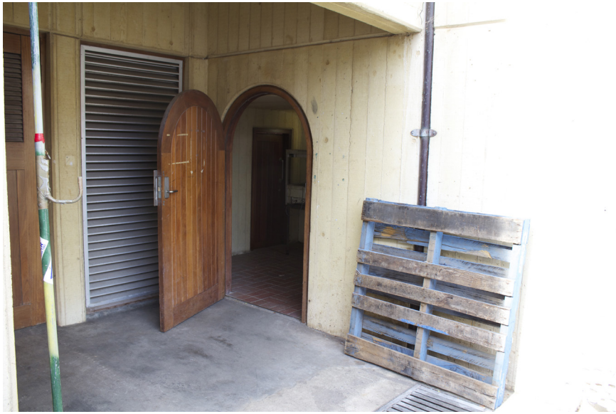
5. Walk through this door and up to the top of the stairs (This building is Cameron Hall)
